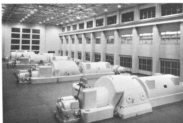
Interior of Russell Station showing all four turbo-generators in operation
